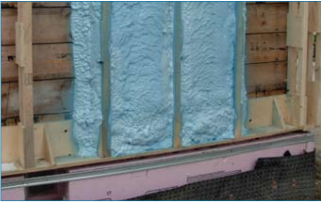
Figure 3 Exterior wall under construction
