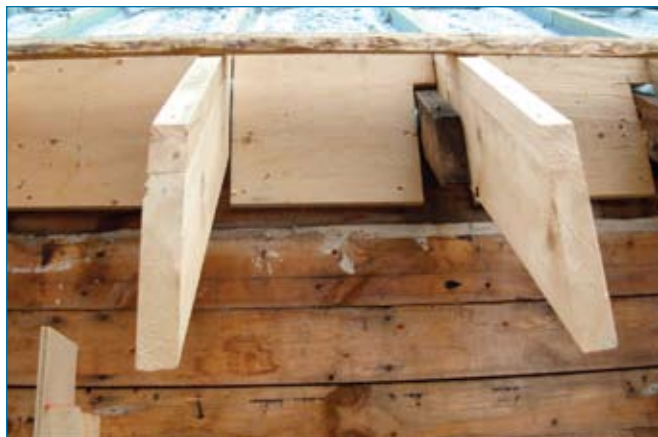
Figure 2 New rafters adjacent to existing rafters
